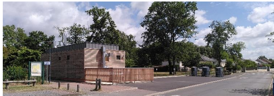
La Ville-aux-Dames, Chaufferie biomasse
